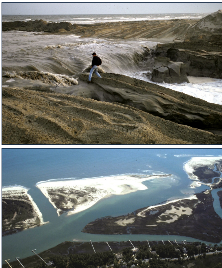
FIGURE T-10. The second relocation of Captain Sams Inlet in April 1996. [UPPER] First tide into the channel basin on 4 April during a rising tide. [LOWER] The new channel (left side) before completion of the closure dike across the old channel.
