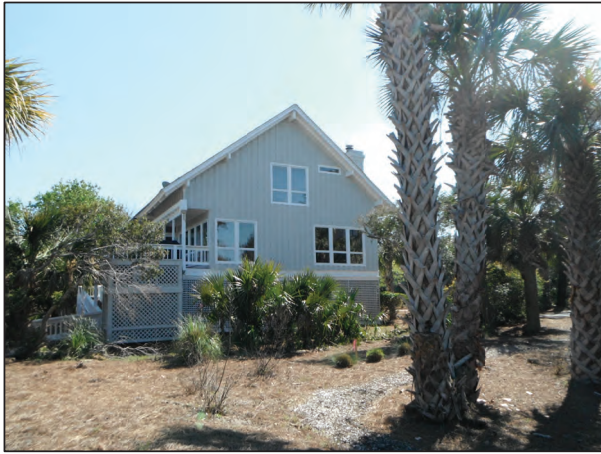
EXISTING SIDE VIEW
