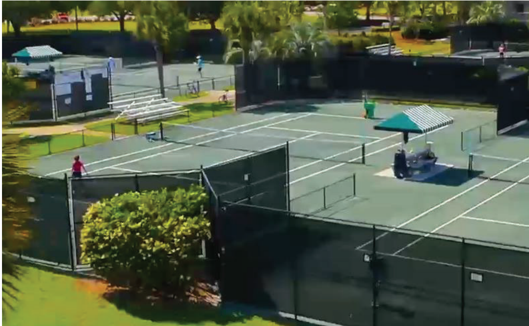
Figure 1 - Fence and Material Photo of the Existing Courts
