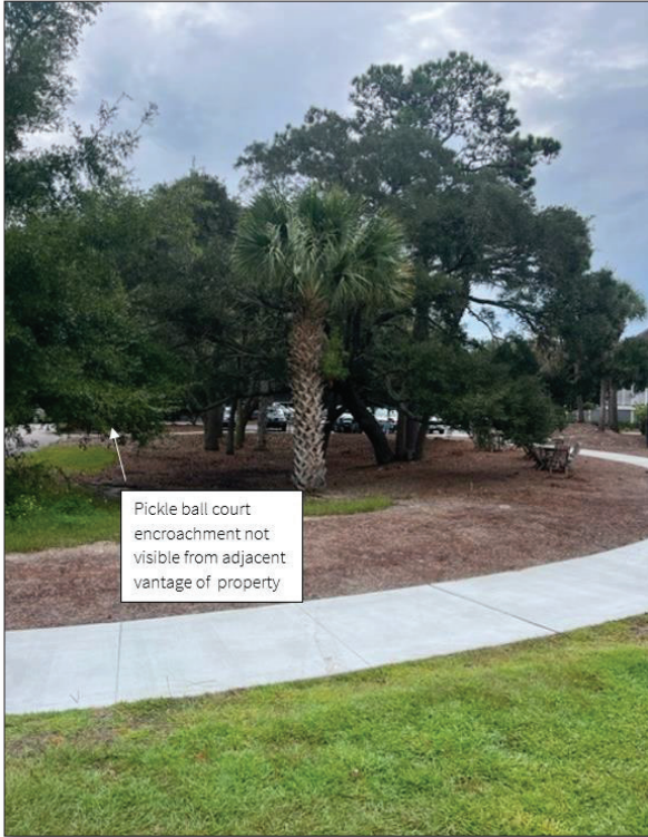
Figure 4 - Pickle ball encroachment from adjacent property
