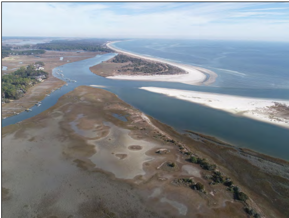
FIGURE 5.1.2I. [UPPER] Volume changes in reach 12 along Kiawah Spit since 2005. The western half of the reach has eroded since 2010, while the eastern half (including the area near the neck of the spit) has accreted. [LOWER] Kiawah Spit at low tide in January 2019. The large dry-sand beach on the down-stream side of the spit suggests it is growing southwest towards Seabrook as the inlet channel migrates down shore.
