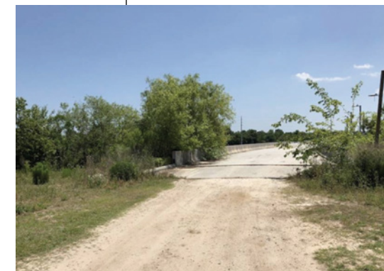
find the pavement ends with nothing but dirt on the other side
