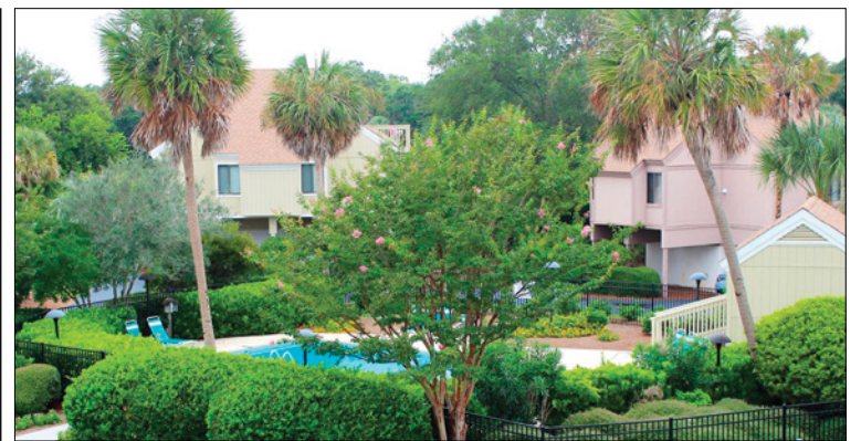
Sealoft Villas - Seabrook Island
