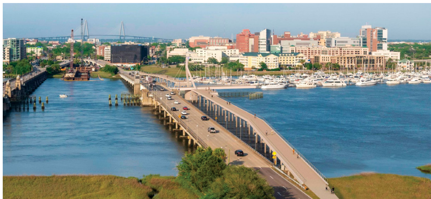
The movable span on the proposed Ashley River Crossing bridge would function as a swing span drawbridge | Renderings by HDR, Inc., courtesy City of Charleston
