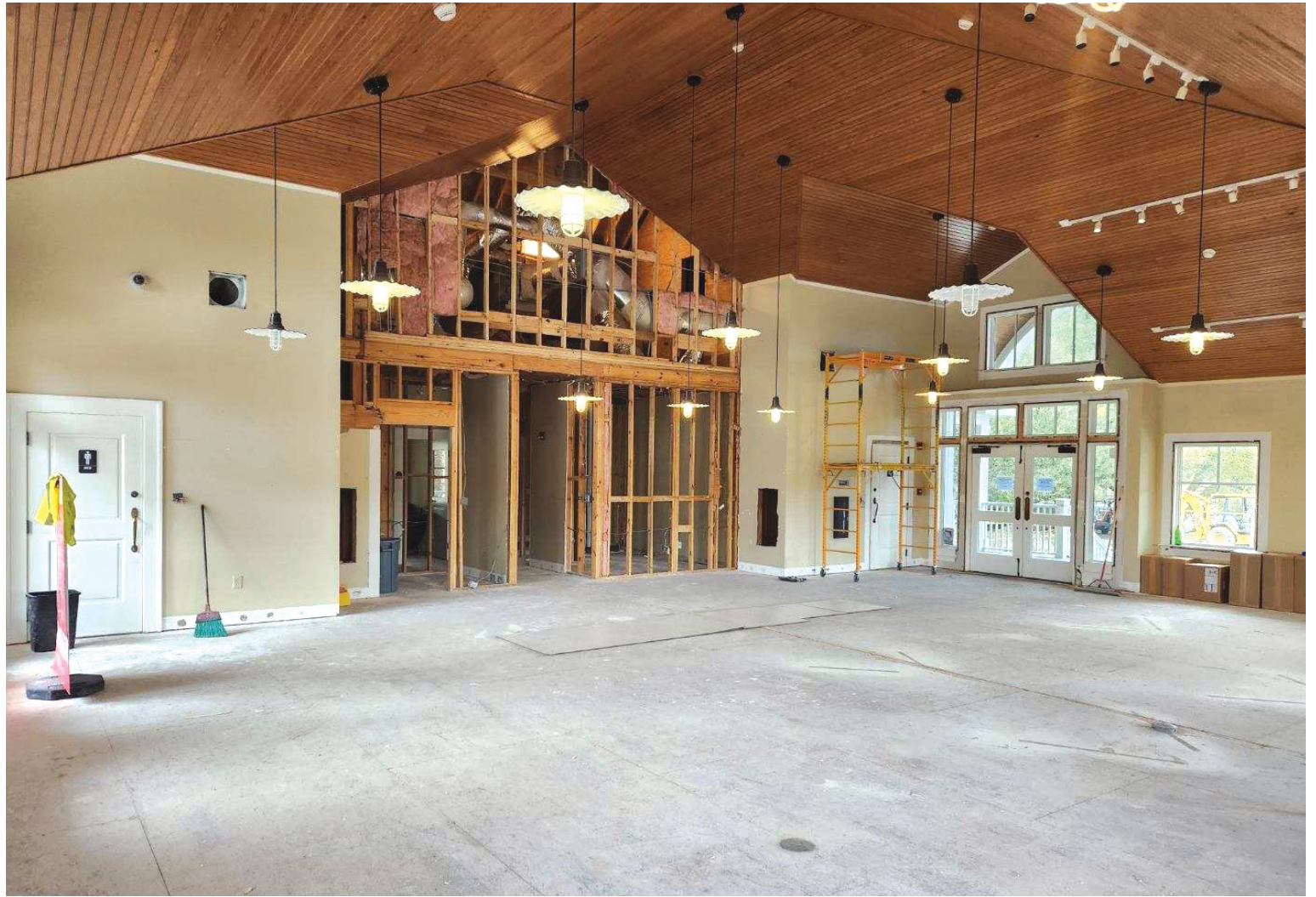
Racquet Sports Pro Shop interior renovation
