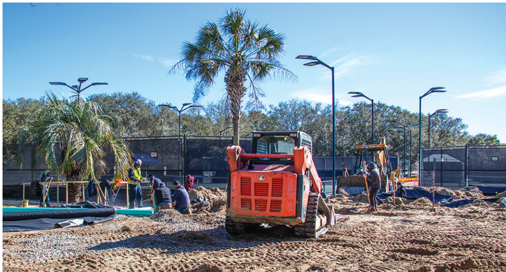
Hardscape and landscape improvements are currently underway.
