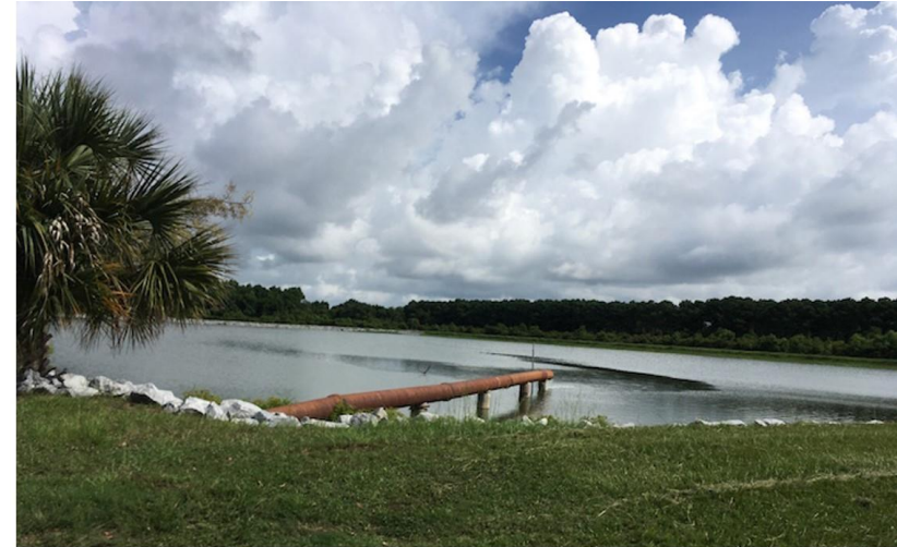
Seabrook Island Utility Commission Water Reservoir Photo Source: Sue Holloman, Tidelines, July 2018.
