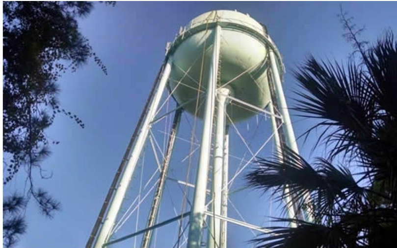
Seabrook Island Water Tower Photo Source: www.louisberger.com
